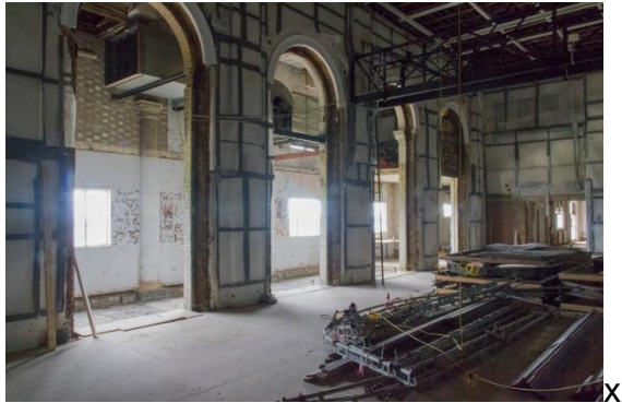
Figure 26. Studio A (August 2019) with arch infills removed and given essential repairs.
